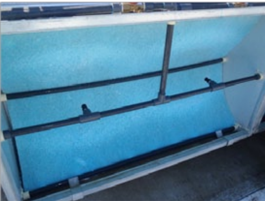
Figure L6: Inside of a current, new FlashCool Nacelle
