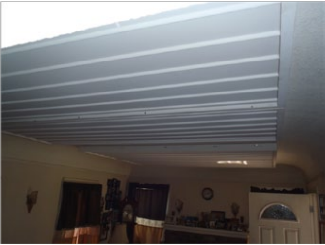
Figure S3: The panels attach directly to the ceiling keeping the installation costs to a minimum (these panels are shown during installation and are still unfinished)
