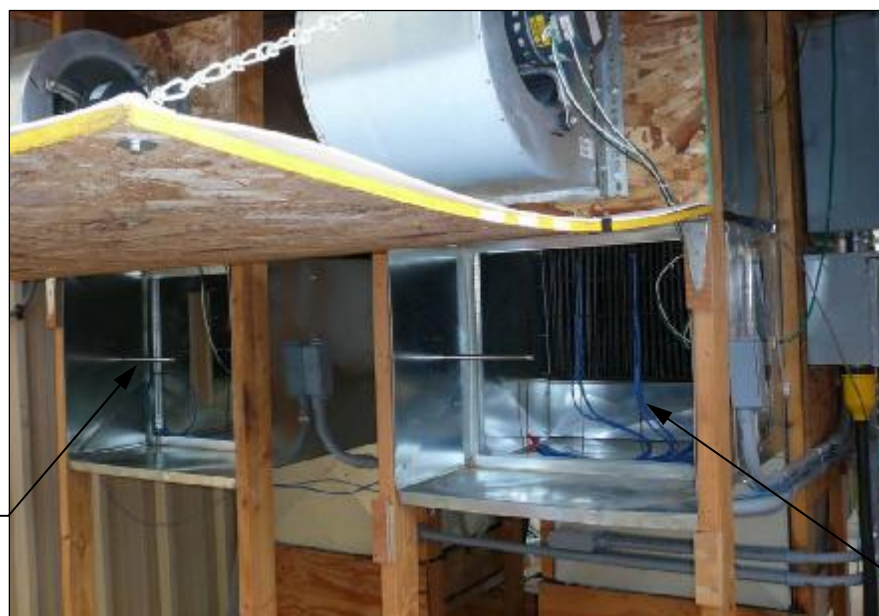
Figure 6 – Instrumentation in Dry Passages
