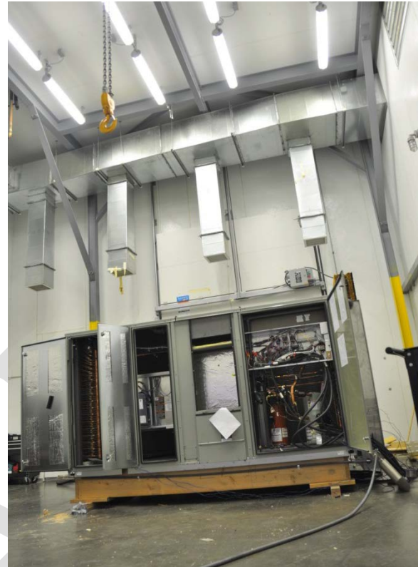
FIGURE 2: TRANE VOYAGER DC DURING SETUP
