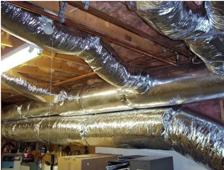
Residential HVAC Ducts
