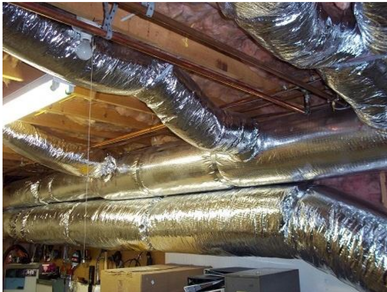
Residential HVAC Ducts
