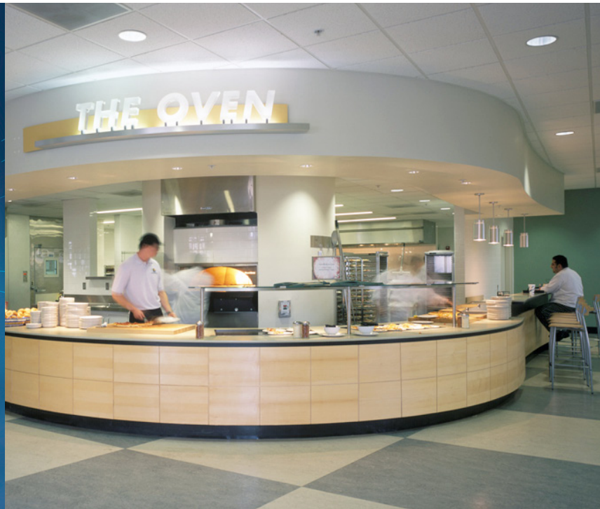
Demand ventilation fan speed controller installed at the kitchen of the Carrillo Dining Commons, University of California, Santa Barbara
