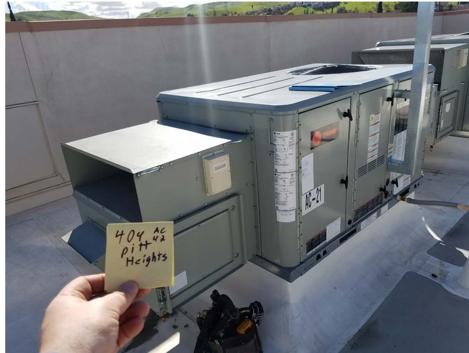
Roof Top Unit (RTU)
