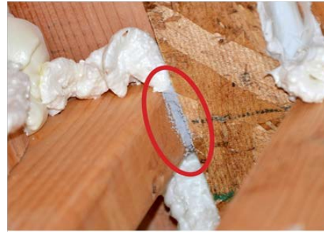
Sealed leak in between manual caulk application at the Honda Smart Home
