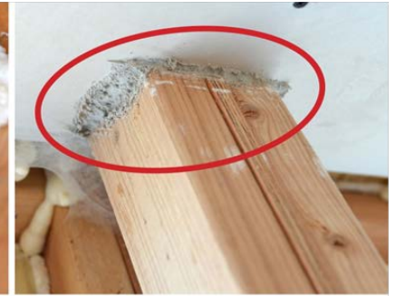
Large sealed leak on a ceiling beam at the Honda Smart Home
