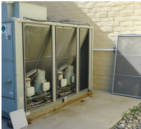
Removal of existing inlet grilles
