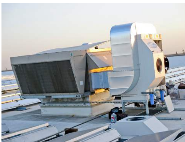
Indirect evaporative retrofit for RTUs
