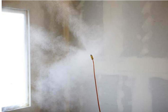
Figure 8. Photo of sealant atomization.
