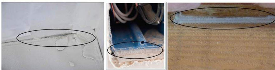
Figure 11. Photographs of envelope leaks sealed during the field tests (sill plate, electrical box, and header).
