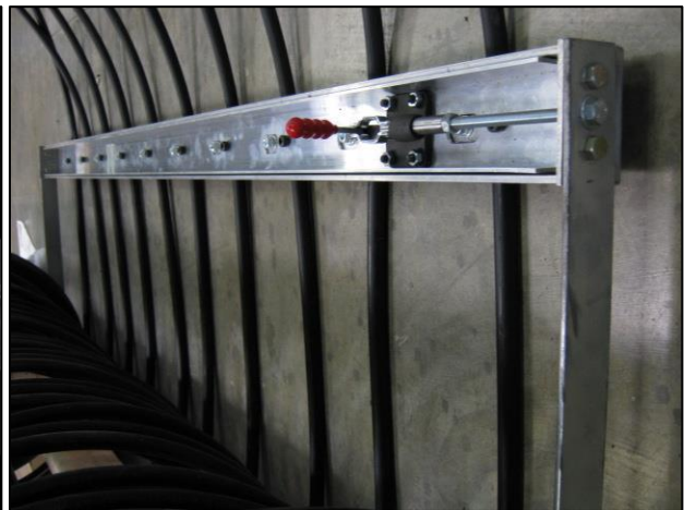
Figure 15 – Aluminum spacer rake guiding HDPE tubes at 6" spacing.
