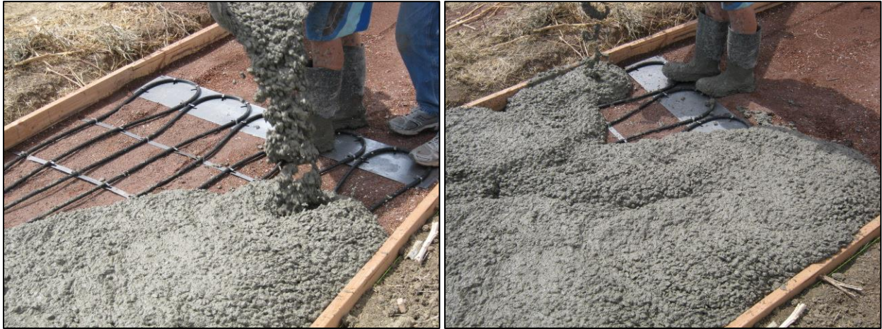
Figure 26 – Pouring concrete over the spacer bars and end plate
