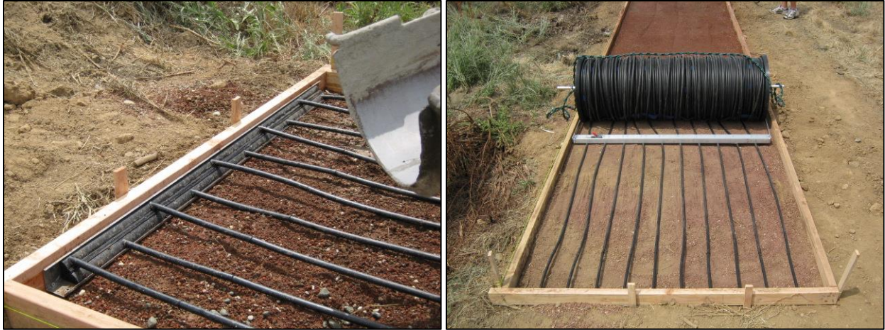
Figure 22 – Securing the manifold at the beginning of the installation (left) and setting up the spool and rake assembly for the rollout (right).
