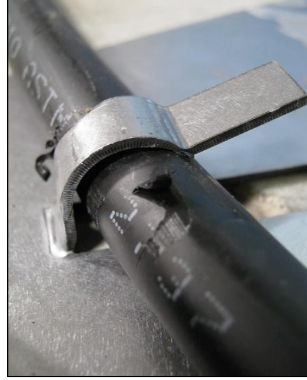
Figure 14 – Return bend stabilization consisting of end plate and two spacer bars with clips punched from sheet metal.
