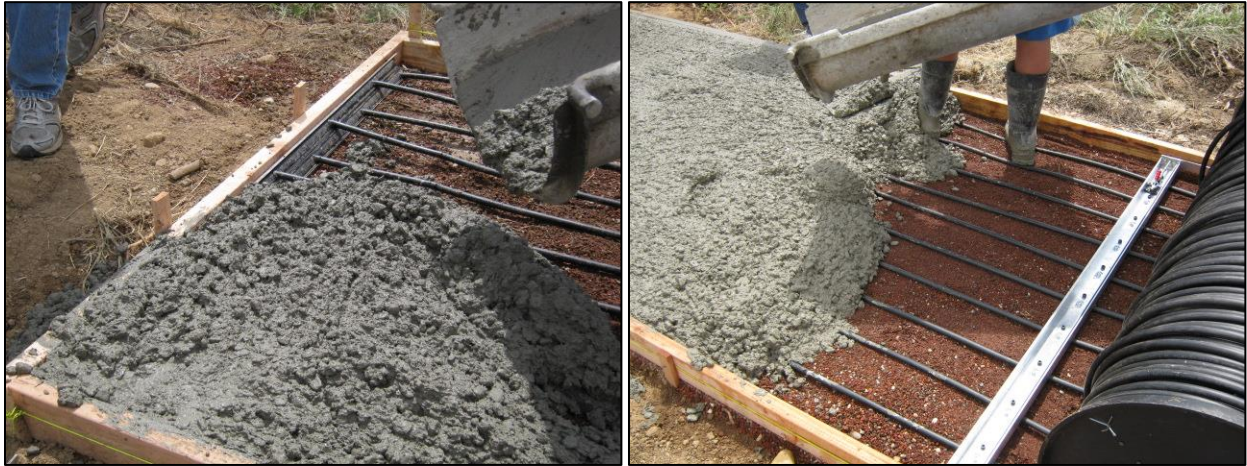
Figure 23 – Pouring concrete onto the manifold and tubes.
