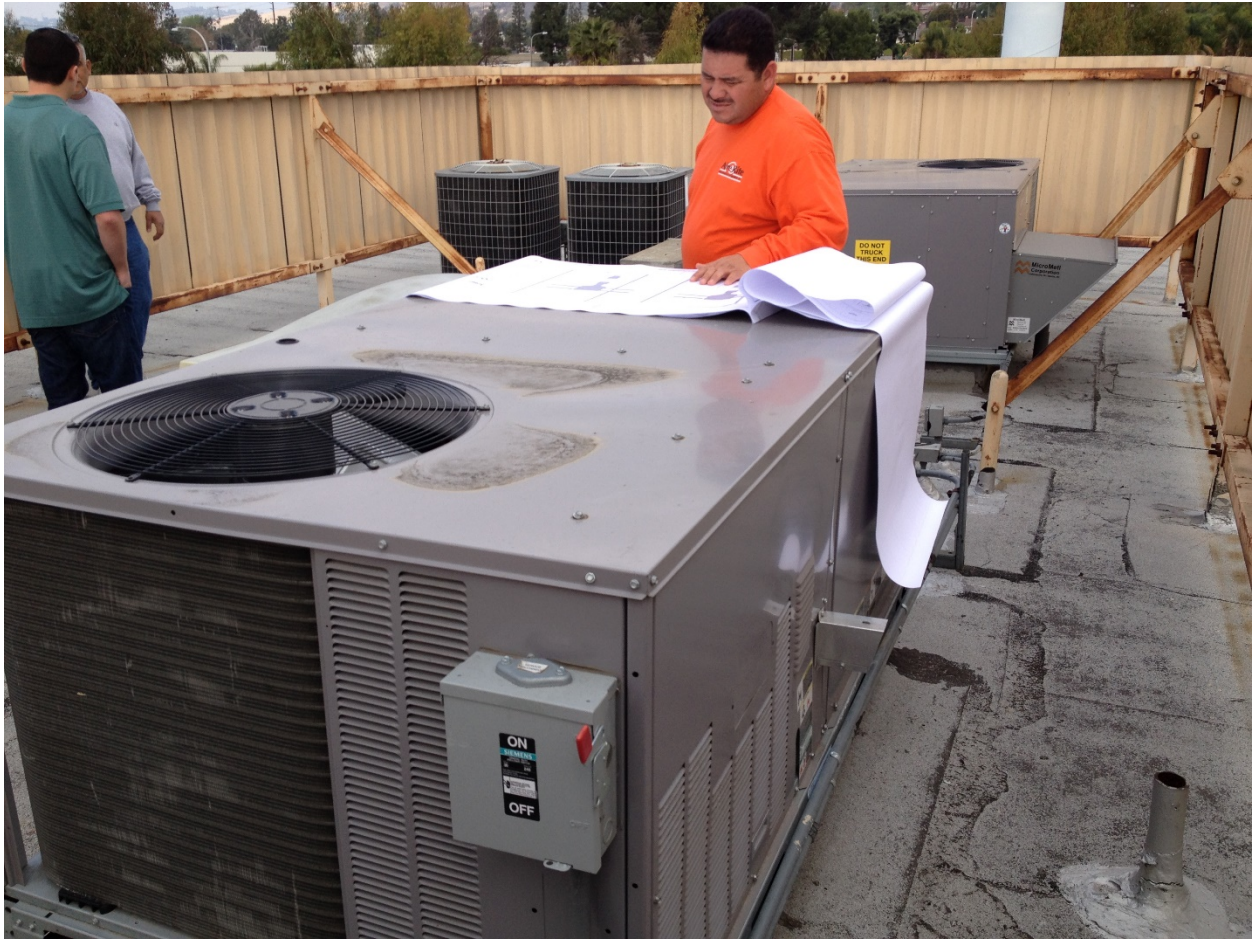
FIGURE 4: RTUs ON THE PLACENTA ROOFTOP
