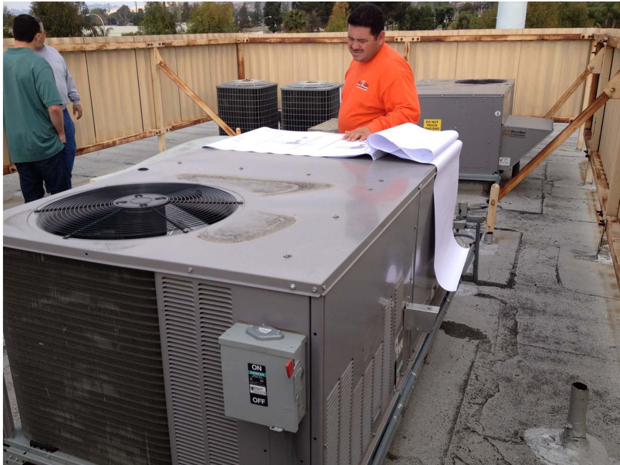
FIGURE 4. RTUs ON THE PLACENTA ROOFTOP
