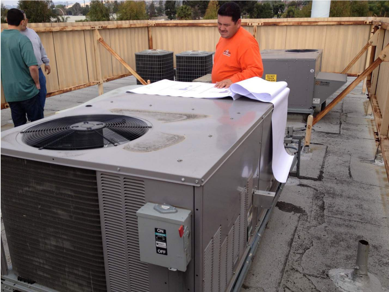
FIGURE 4. RTUs ON THE PLACENTA ROOFTOP
