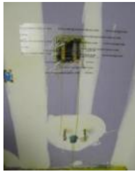
Figure 29. Tape on large penetration in bathroom wall to protect plumbing elements
