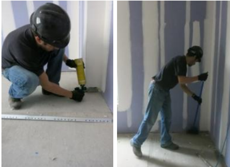
Figure 5. (L) Sealing large holes with foam; (R) sweeping debris for sealant access
