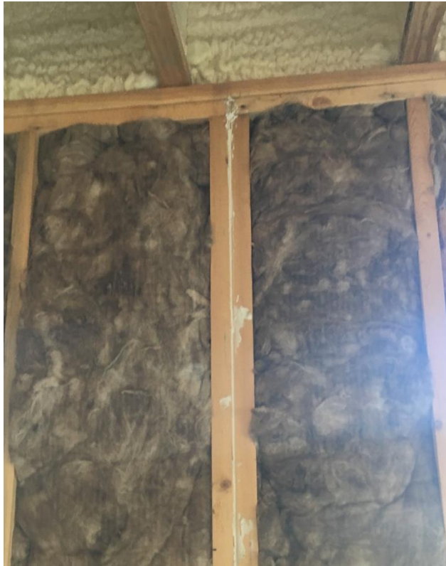
Caulk at seams where wood is joined
