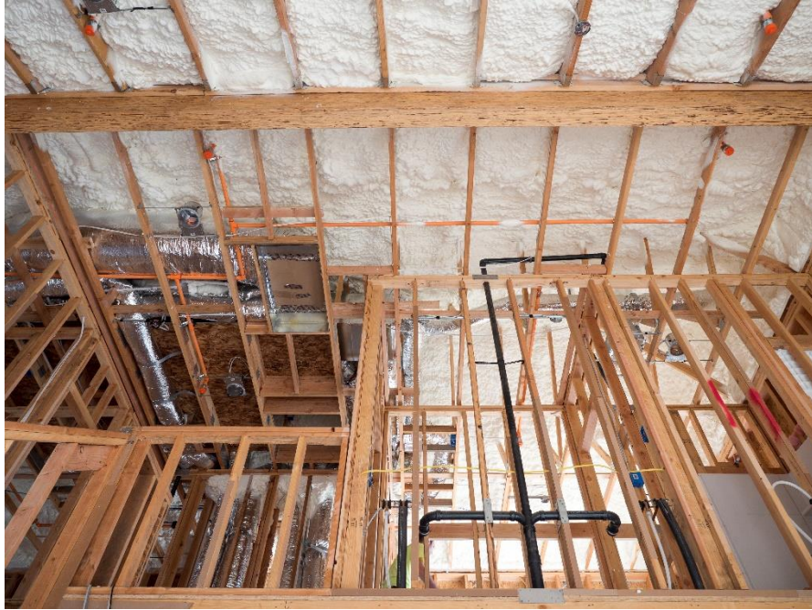
Foam at roof deck
