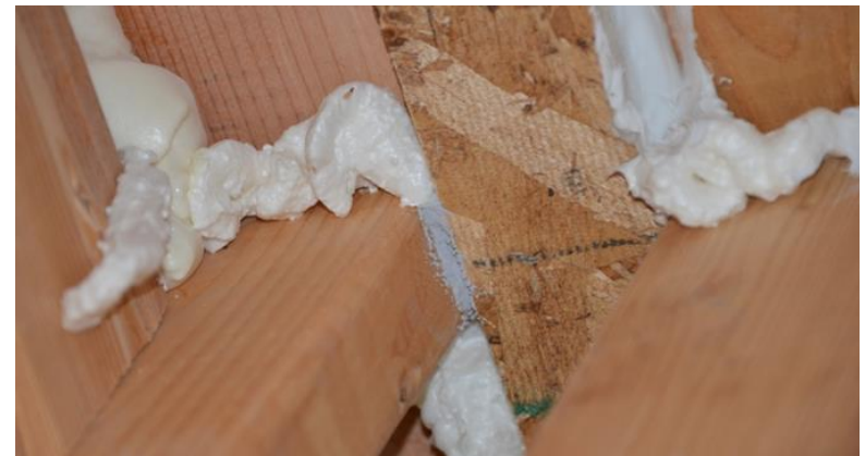
Seal formed between gap in foam
