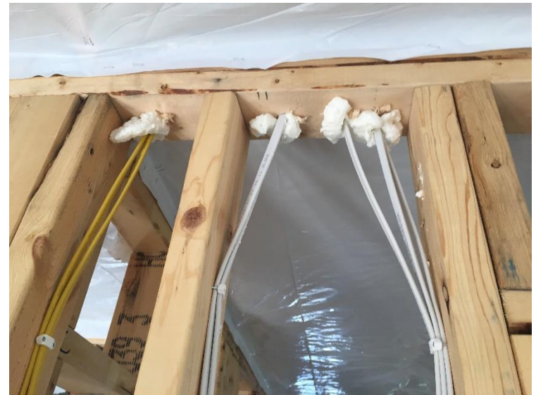
Can foam at wire penetrations
