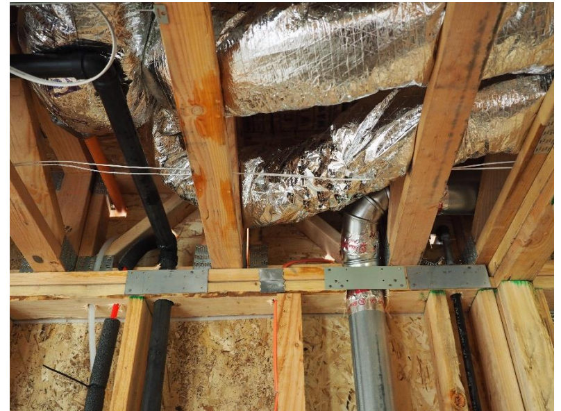
Rim joist penetrations
