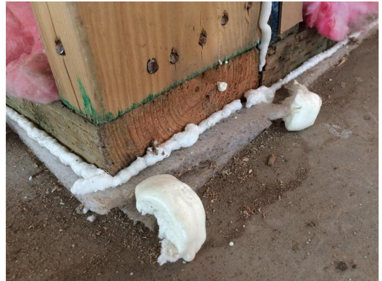
Can foam and gasket at sill plate
