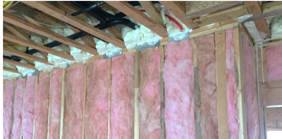
Foam at rim joist
