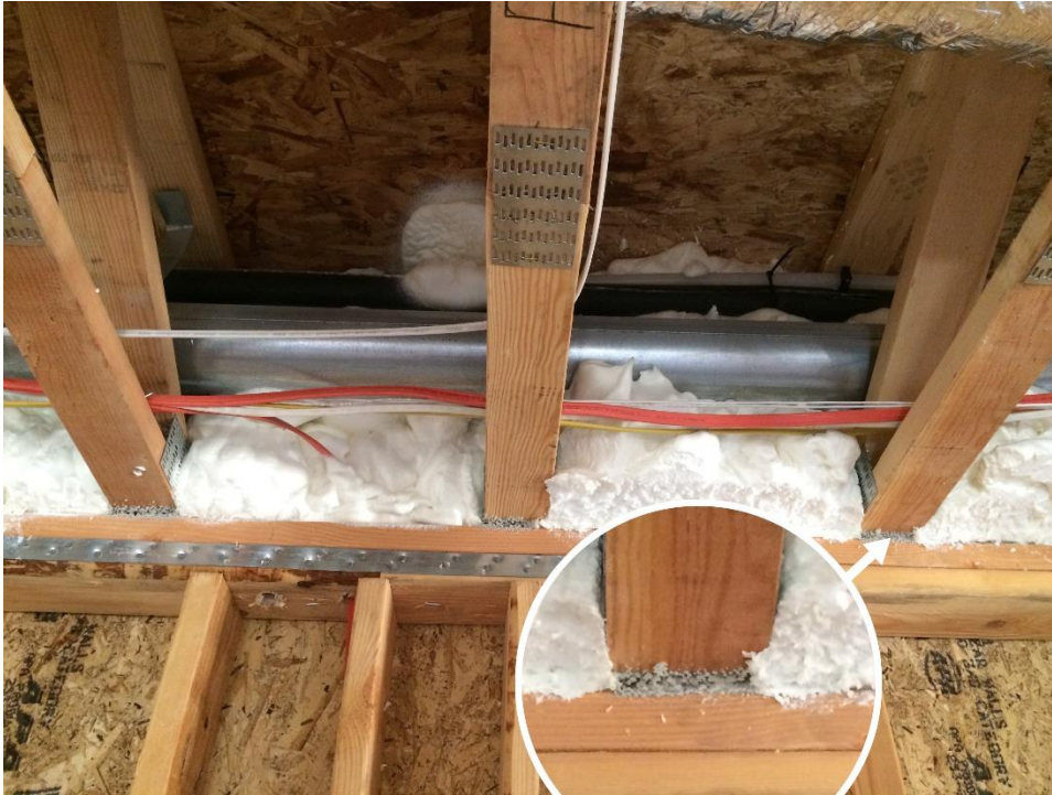
Seals formed under trusses
