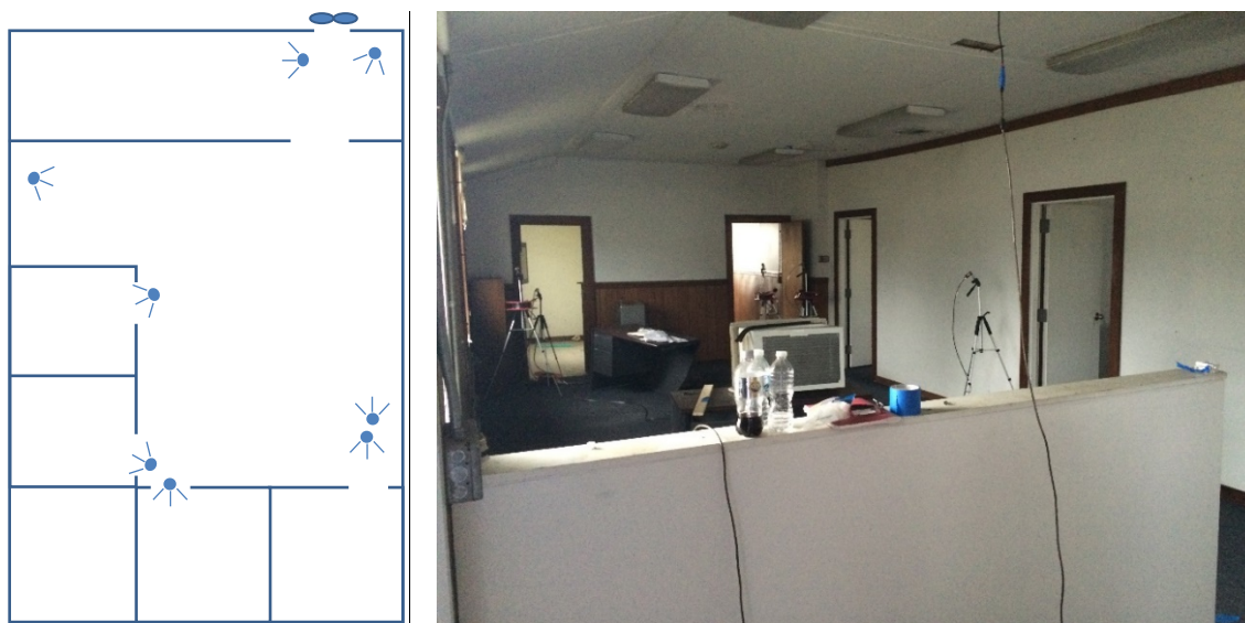
Figure 21. Nozzle Arrangement during Sealing in A5436 (left) and Photo of Nozzle Setup (right)
