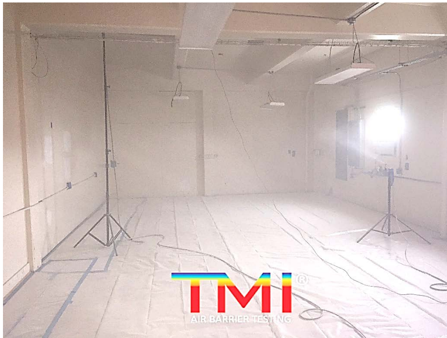
Figure 18. Building 2177 at Quantico Prepped for Aerosol Envelope Sealing
