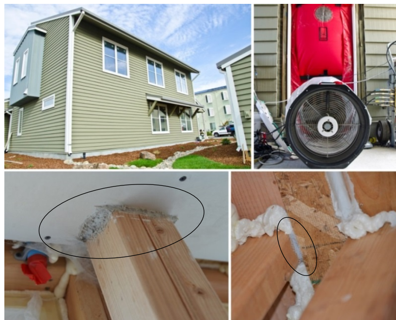
Figure 2. Photos of Aerosol Sealing Installation on Single-family Home Including Examples of Seals Formed.
