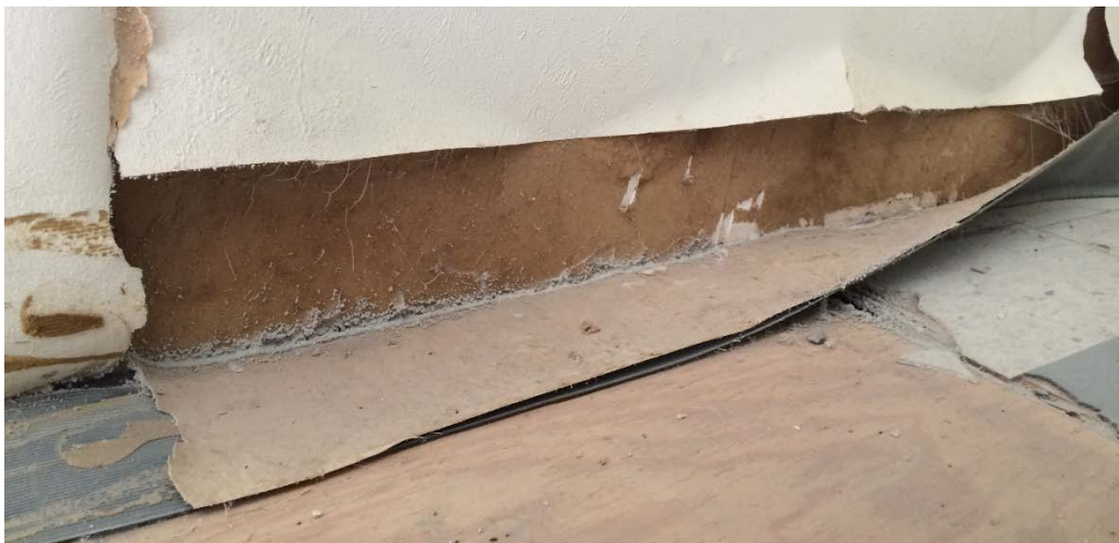
Figure 24. Photo of a Seal Formed at Baseboard of Building A6372 at Fort Bragg Army Base
