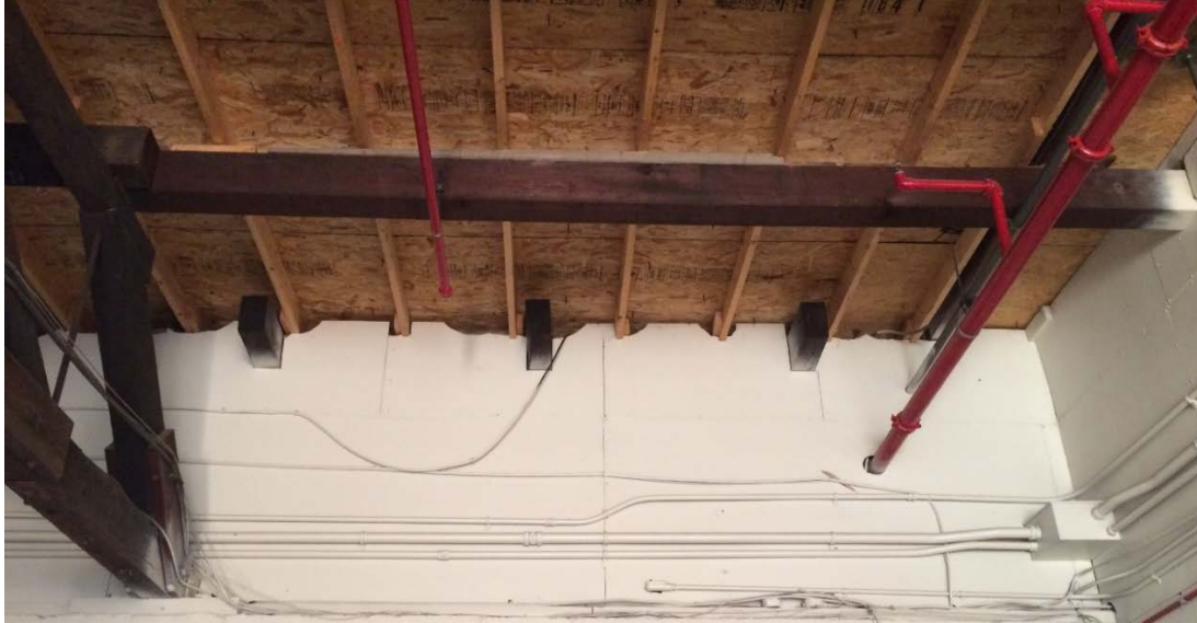
Figure 26. Photo Showing Large Holes in Wallboard at the Roof Rafters of Building M/608A at NSA Mechanicsburg
