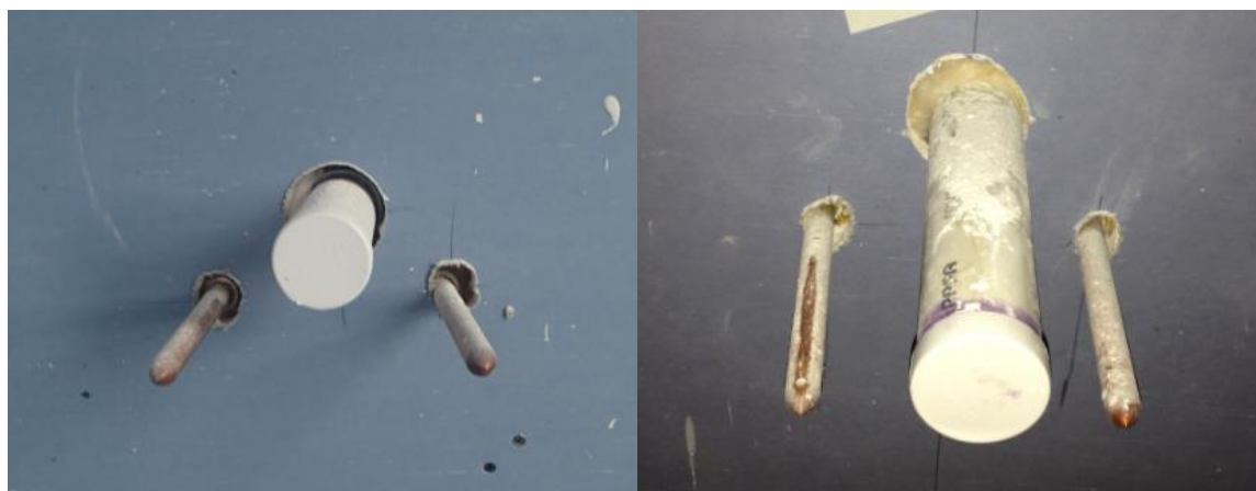
Figure 60: A gap in the floor to wall detail too large for aerosol to seal before pre-sealing work (left) and after a mineral wool backing material was applied (right)
