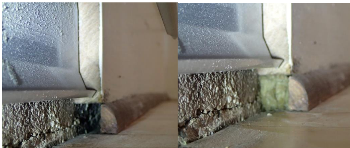
Figure 60: A gap in the floor to wall detail too large for aerosol to seal before pre-sealing work (left) and after a mineral wool backing material was applied (right)
