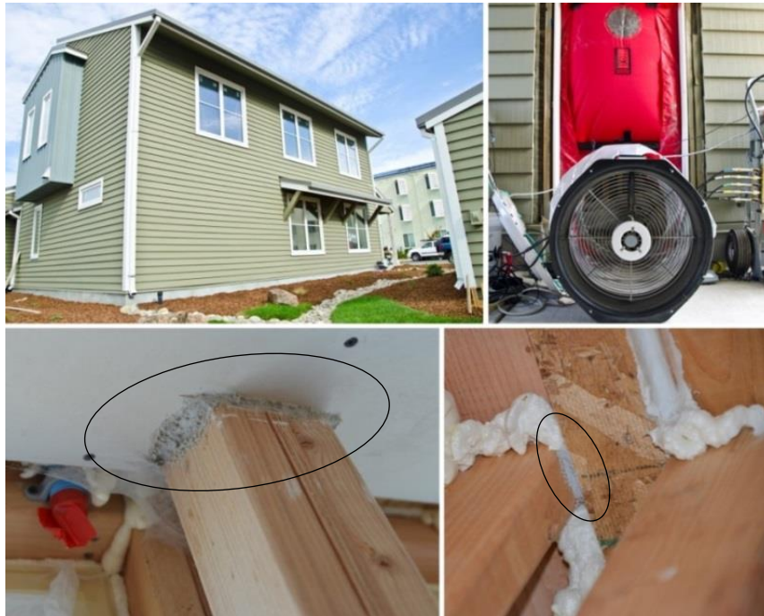
Figure 11: Photos of Honda Smart Home before aerosol envelope sealing application
