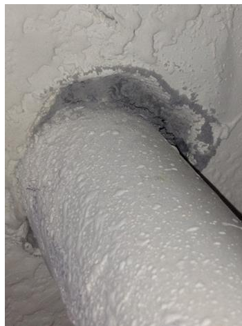
Plastic pipe through ceiling
