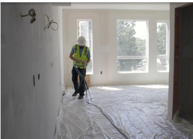
Figure 3. Image of air sealing process in the field
