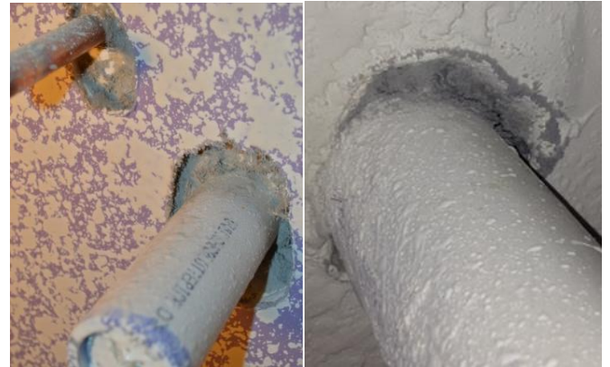
Figure 2. Visual images of sealed air leaks
