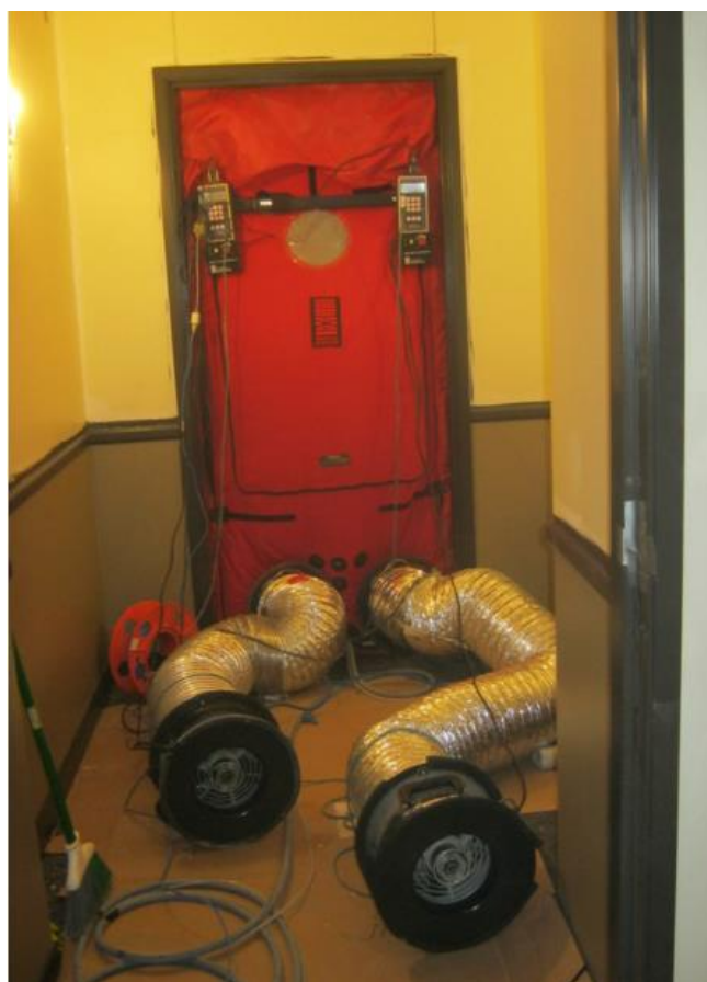
Figure 64: Photo showing flexible duct used to separate blower door fan from the frame
