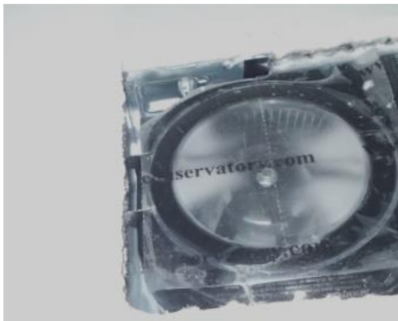
Figure 58: Shower handle temporarily sealed to protect moving parts and intentional leaks from being sealed
