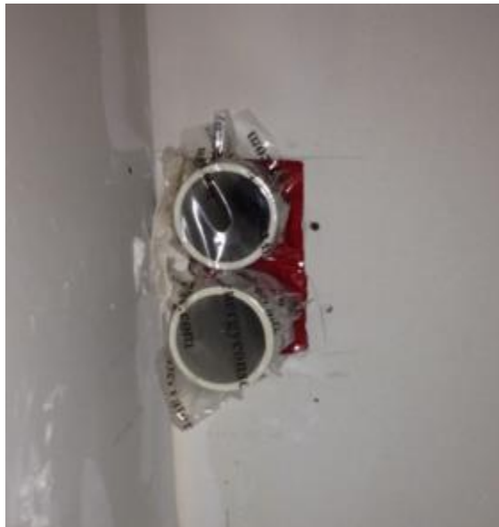
Figure 56: Temporary sealing of HVAC combustion air and exhaust penetrations
