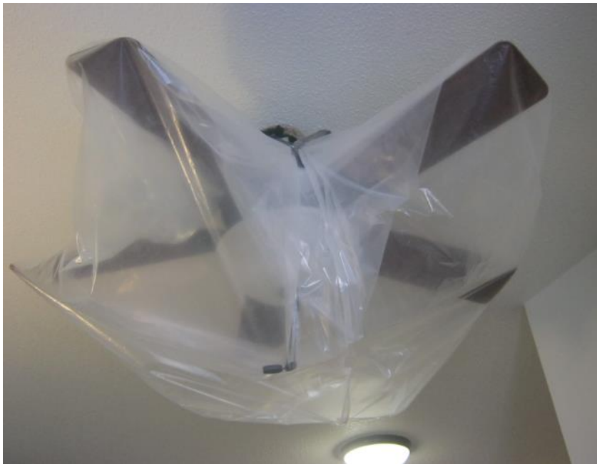
Figure 55: Protection applied to a ceiling fan prior to air sealing work
