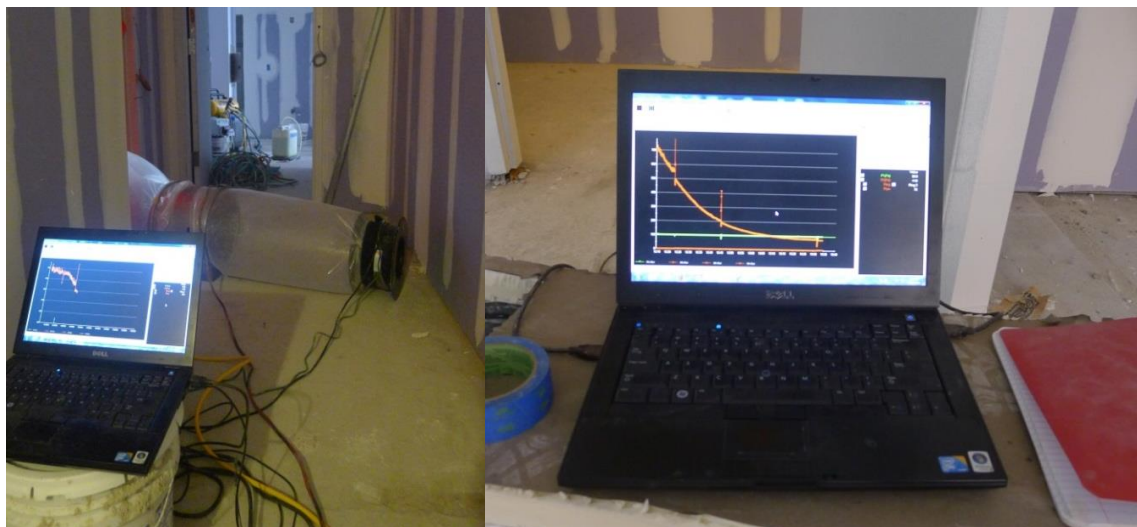
Figure 14: Photos of software used to track and record the sealing process in real-time
