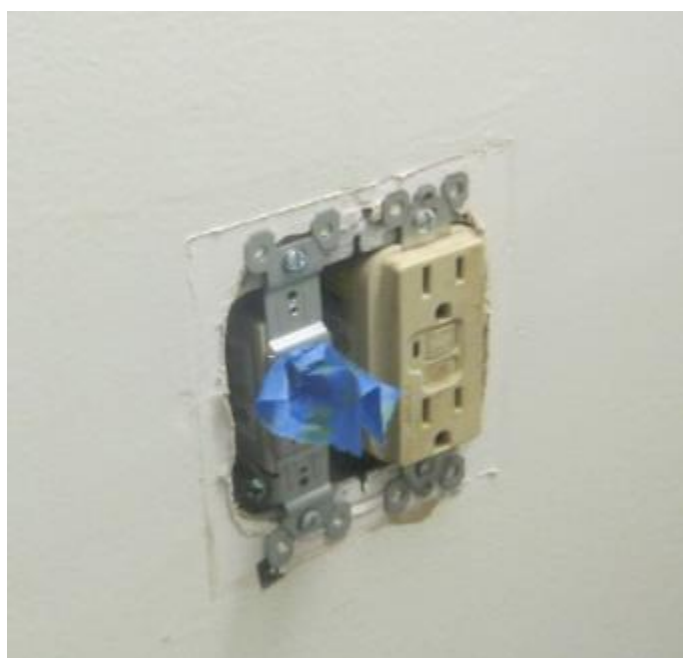
Figure 63: Outlet covers were removed from electrical outlets to allow aerosol sealant better access to leaks inside the electrical boxes
