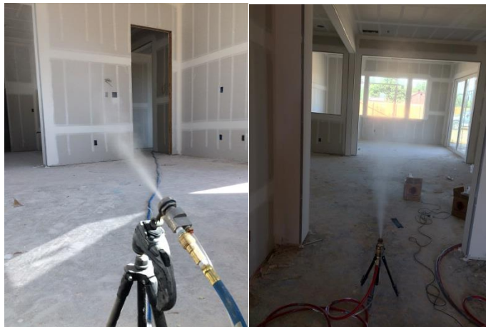
Figure 52: Sprayer direction checked before sealing starts
