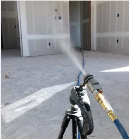
Emitters are placed throughout the house to inject an aerosol into the air while pressurizing the house.
