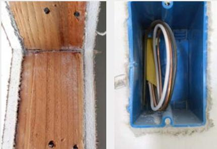
The aerosol collects at gaps in the building and gradually seals leaks.
